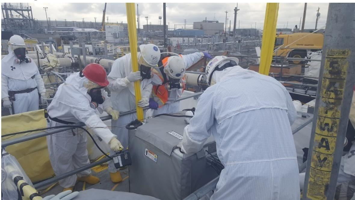
*Workers with Hanford Site tank operations contractor Washington River Protection Solutions install remotely operated, specialized equipment to retrieve waste from single-shell tank AX-103 at the Hanford Site.*
