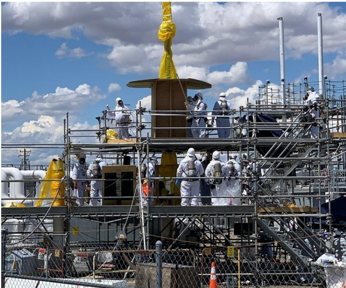
*To prepare decades-old tanks for efficient and safe waste retrieval operations, workers remove old systems and equipment, like this thermocouple that was used to measure the temperature of waste. They install new retrieval and monitoring equipment, ventilation safety systems, and waste transfer lines.*
