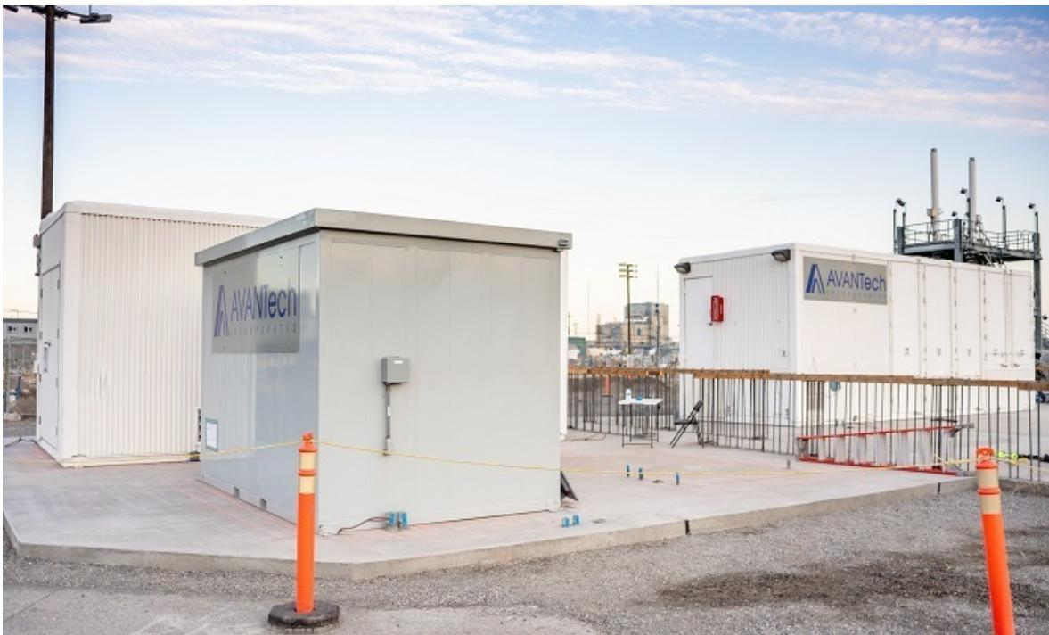
From left, auxiliary, control, and process enclosures for the Tank-Side Cesium Removal system, critical to the Direct-Feed Low-Activity Waste approach at the Hanford Site, have been anchored to a concrete pad next to large underground waste tanks in the AP Tank Farm.
