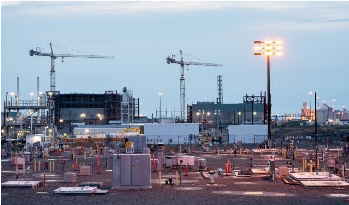
*The white enclosures of the Tank-Side Cesium Removal system are visible adjacent to the Hanford Site's AP Tank Farm. In the background is the Waste Treatment and Immobilization Plant, where waste pre-treated by TSCR will be heated to 2,100 degrees Fahrenheit, mixed with glass-forming materials, and poured into stainless steel containers for disposal.*
