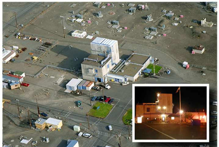
242-A Evaporator and surrounding area
