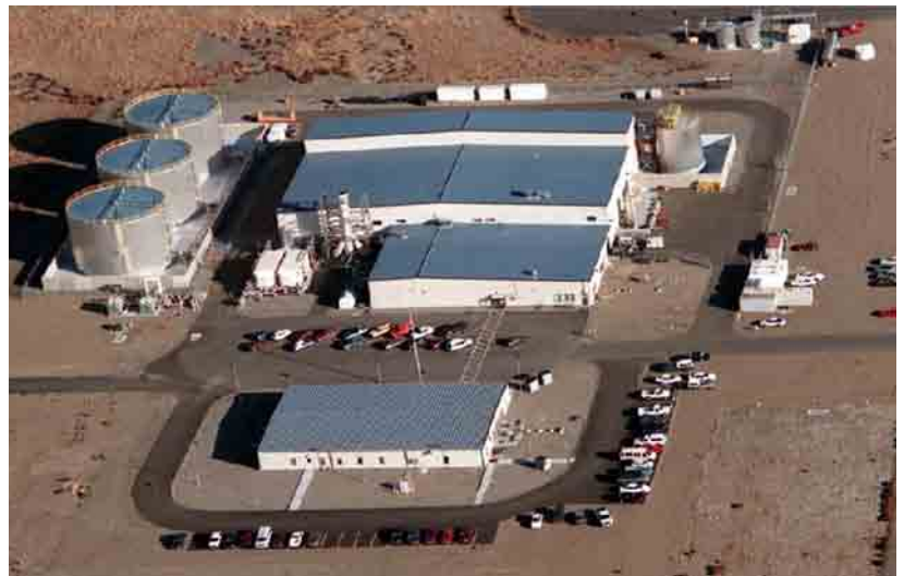
The existing 200-Area Effluent Treatment Facility will be upgraded to treat WTP secondary waste.
