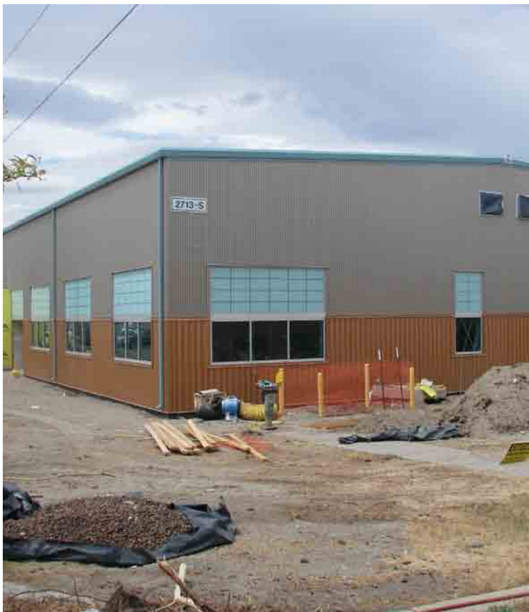
New 222-S Laboratory office building.
