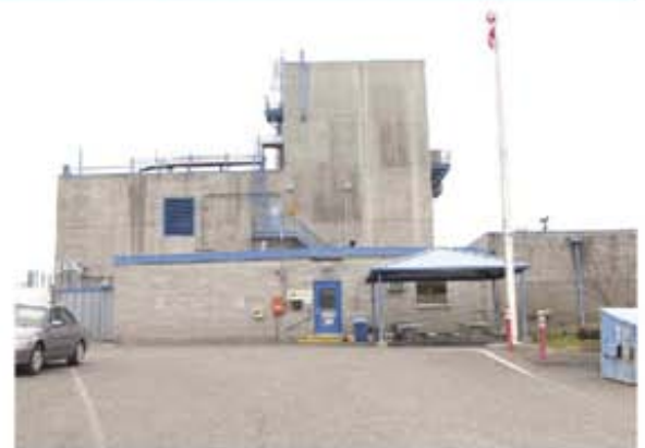
Following a series of upgrades and improvements the 242-A Evaporator resumed operations reducing the volume of waste stored in Hanford's double-shell tanks. This creates additional storage space for waste transferred from aging single-shell tanks and avoids the time and cost of building expensive new storage tanks.
