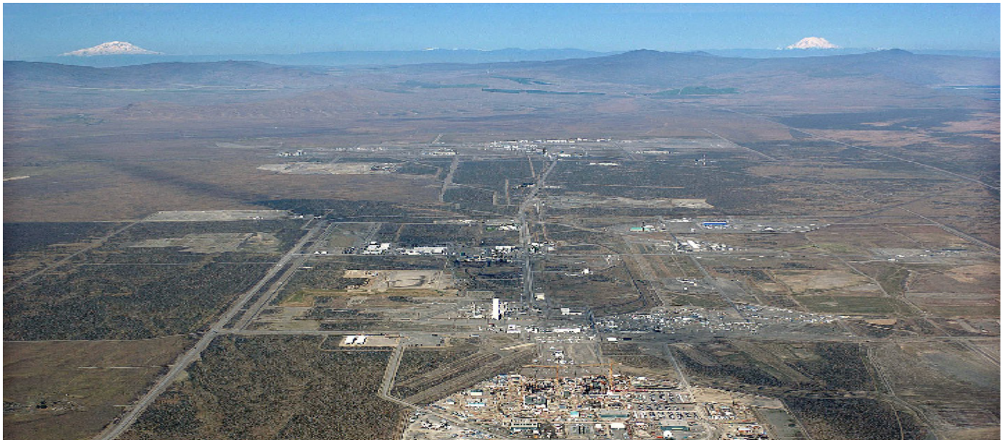
Aerial view of the Hanford central plateau where 177 underground radioactive waste storage tanks are located near the center of the 560 square-mile Hanford Site.
