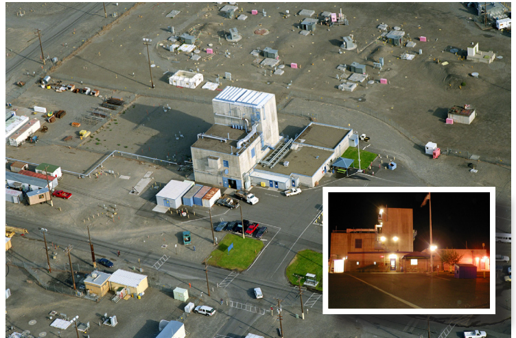
242-A Evaporator and Surrounding Area
